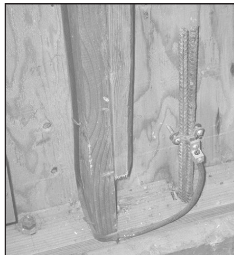
Figure 5 — Typical Ufer Ground
